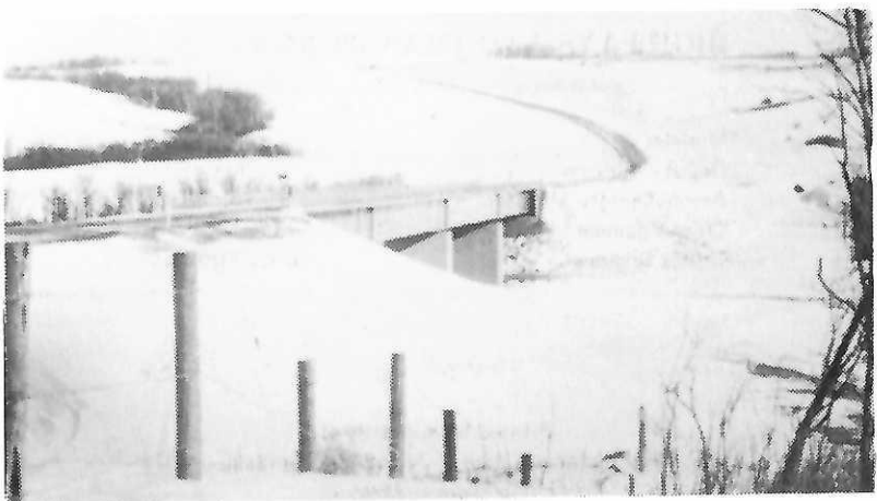
THE NEW BRIDGE - COMPLETED
